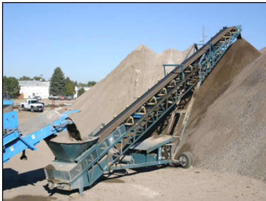
Figure 5. Example of aggregate processing facility.
