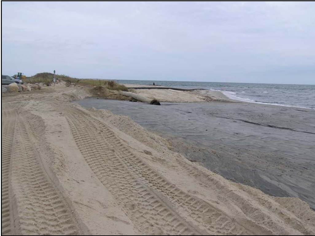
Figure 2. Example of hydraulically placed beach nourishment on the south shore of Cape Cod, Falmouth, MA.
